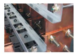
^ Applying a mark (paint, brittle coating) will show any loosening and can also be used to check that tightening has been carried out correctly (tell-tale)
