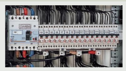
Phase 1 supplies: 2 DX 32 A, 2 DX 20 A, 1 DX 10 A Phase 2 supplies: 1 DX 32 A, 2 DX 20 A, 3 DX 10 A Phase 3 supplies: 1 DX 32 A, 3 DX 20 A, 1 DX 10 A
