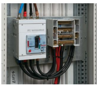
^ For the supply end of medium power distribution panels, the 250 A modular distribution block Cat. No. 048 77 can also be fixed on a plate
